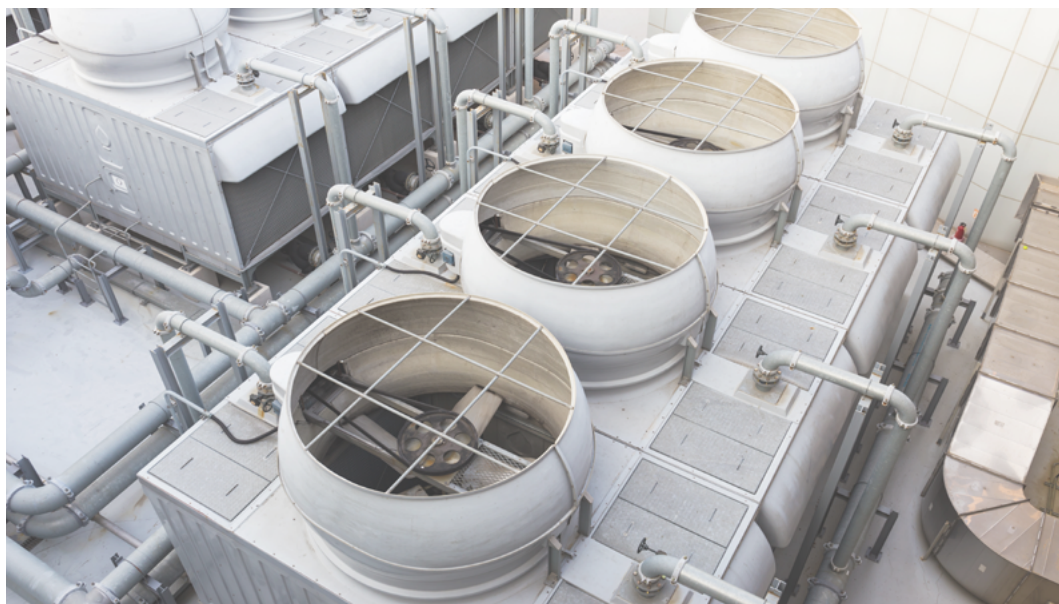
The microorganisms present in cooling and process water like to set up home in cooling towers, creating a biofilm that gradually clogs the system. Concentrated hydrogen peroxide can be used for longer-term cleaning and maintenance cycles in cooling tower systems.
