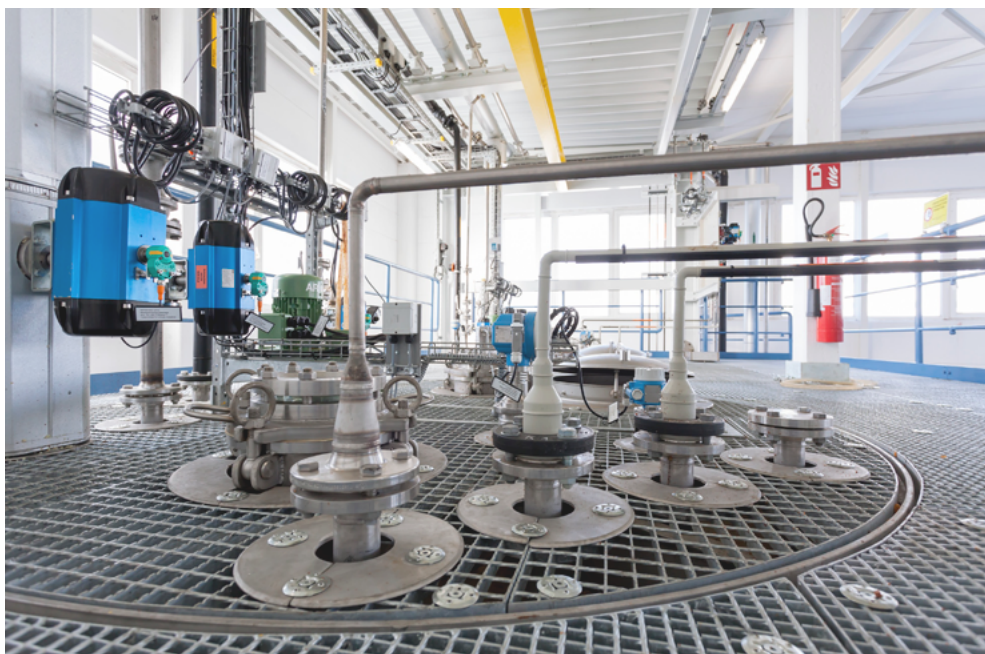
A wastewater treatment plant that uses Eisenmann's proprietary, two-reactor Fenton's reagent-based process called Fentox. EISENMANN
