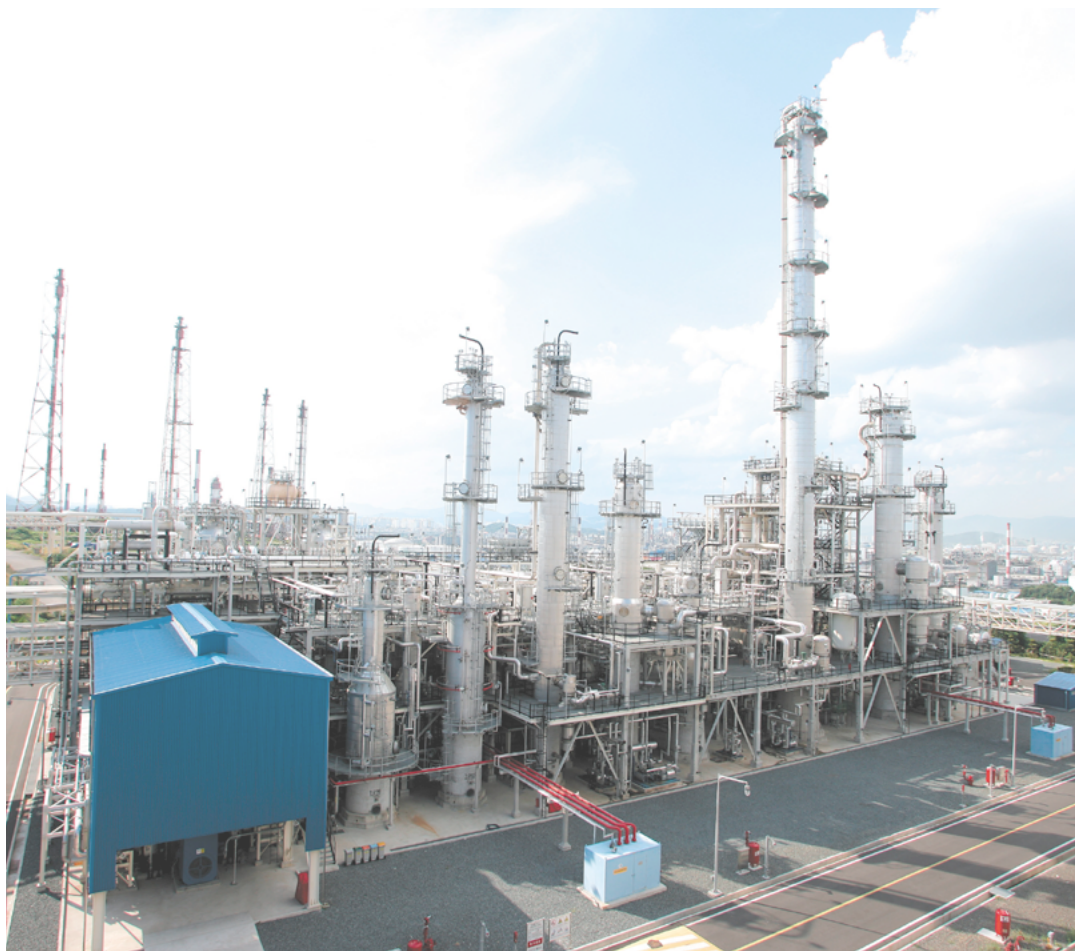
HPPO plants are typically built right next door to a hydrogen peroxide plant, so that the oxidant can be piped directly 'over the fence' for the clean, green production of propylene oxide. EVONIK
